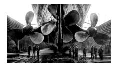
RMS Titanic had three enormous screw propellers to drive it through the water. However, the very first steam ships would have had paddles instead of propellers.
