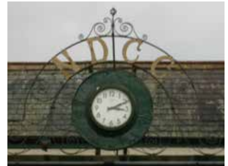
Detail of the pavilion clock.
