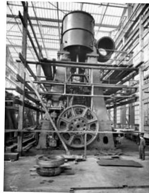
End view of Titanic port main engine near completion in engine works erecting shop, May 1911. © National Museums Northern Ireland Collection Harland & Wolff, Ulster Folk & Transport Museum.
